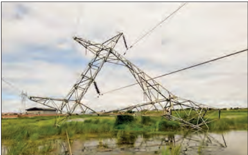
The 132-kV Shwesayan-Tagundine power line was mined down to the ground.
