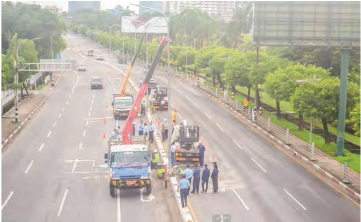
The installation of lamp posts is in progress on Pyay Road.
