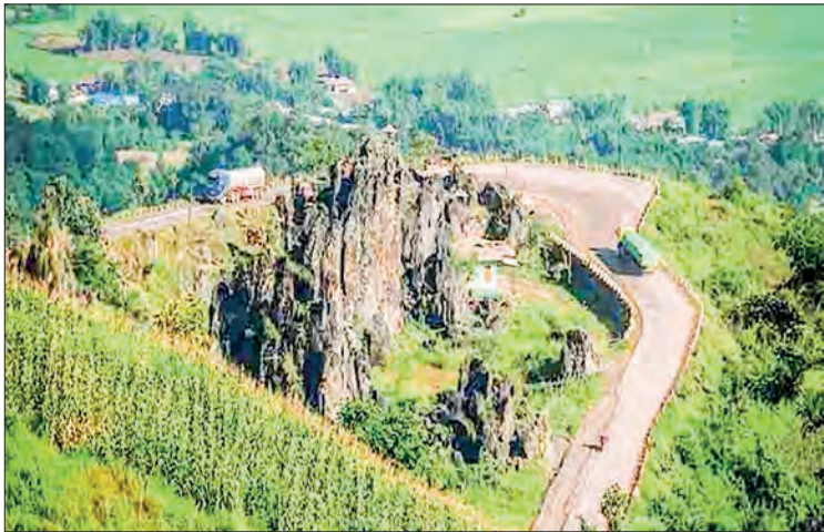
A motor road section in Muse-Mandalay highway.
