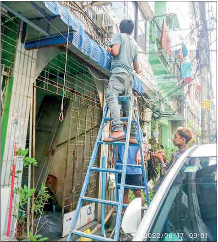
Technicians are seen installing smart meters.
