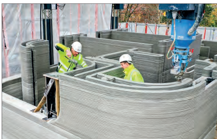
Construction workers stand in the scaffolded construction site of a house, where several layers of concrete have already been applied by a 3D printer, and the next printing stage is already underway, in Beckum, western Germany, on 26 November 2020. PHOTO: INA FASSBENDER / AFP
