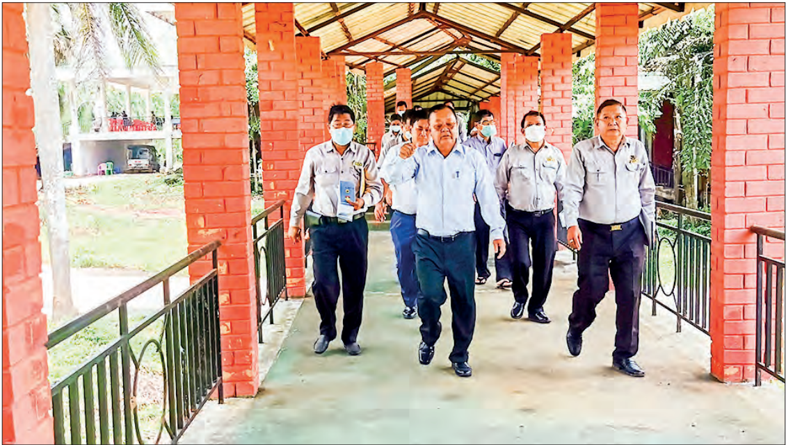
MoC Deputy Minister U Win Pe and party inspects the repair work of the Pyidaungsu Hall on 10 June.
