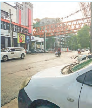
(Left)The Yangon-Dala suspension bridge under construction. (Right) Yangon-Dala ferry services.
