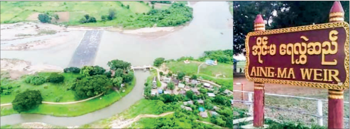
An aerial view of the Aing-Ma Weir.
