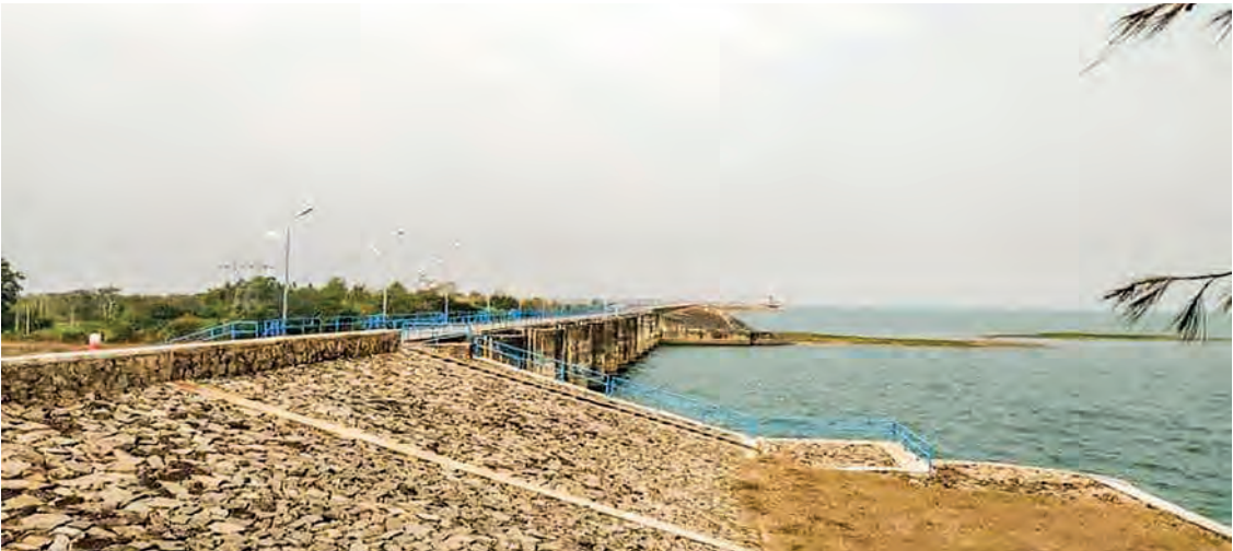
Thaphanseik Dam mainly retains water and releases water into the riverbed of Mu. Then, the irrigation is distributed through the Kintat diversion weir to 170,000 sowing acres.
