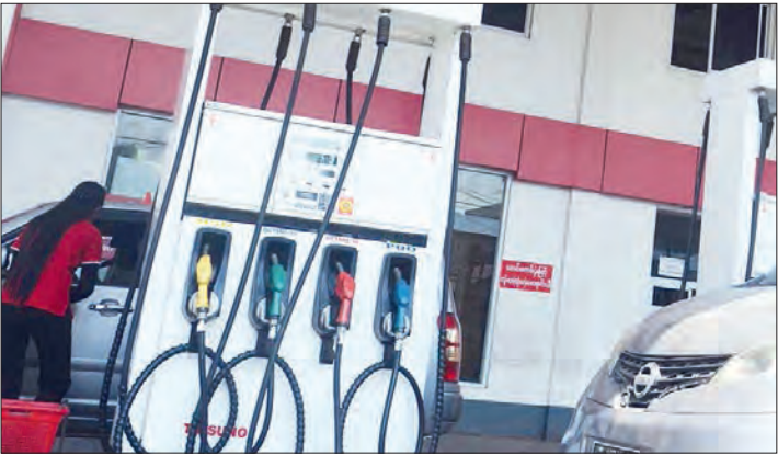
One of the pump stations in Yangon.
