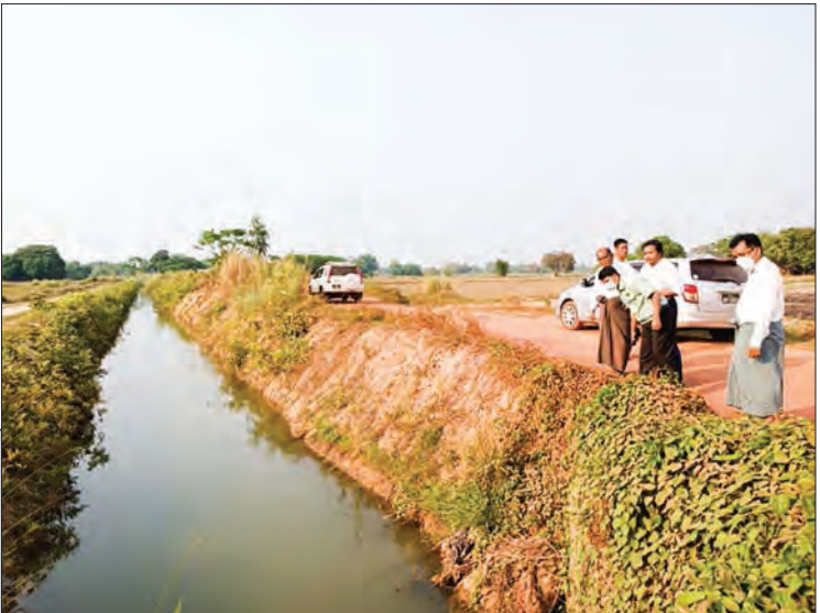
Officials of Bago Township inspect improvement of feeder canal in Bago Township 1 April.
