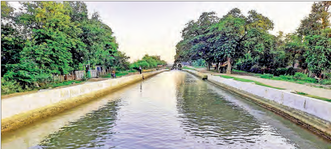
The department annually delivers irrigation water efficiently to farms in the township through the Mezali diversion weir, ensuring an adequate water supply.
