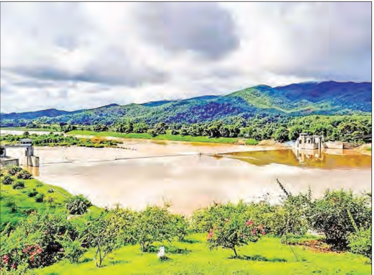
Photo shows the view of the Mezali Diversion Weir.
