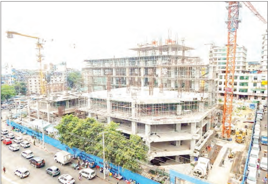
Construction site of New Mingala Market. PHOTO : SOE MYINT AUNG
