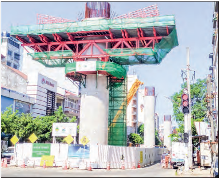
File photo shows Myanmar-Korea Friendship Bridge (Dala) seen under construction. PHOTO: MYINT MAUNG KYAW
