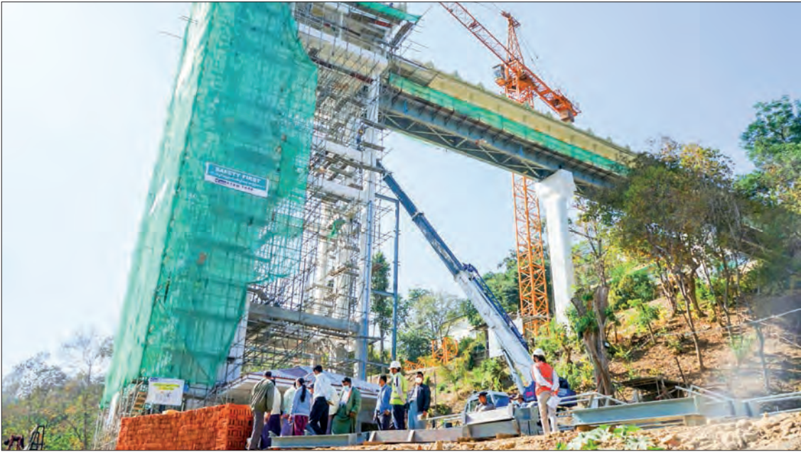
A lift tower is under construction at Mann Shwesettaw Pagoda in Minbu Township with the use of heavy machinery.
