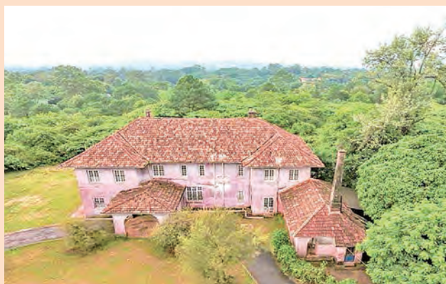
Cherry Myaing: before renovation.
