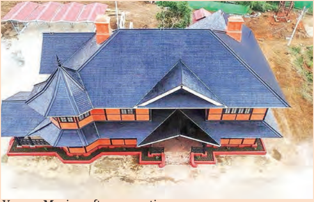
Yuzana Myaing: after renovation.
