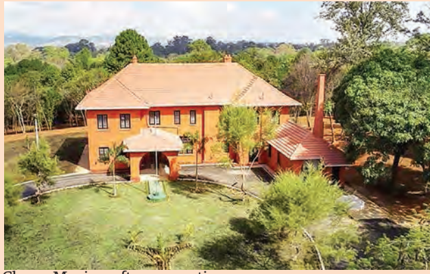
Cherry Myaing: after renovation.
