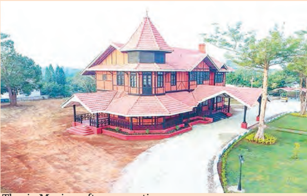
Thazin Myaing: after renovation.
