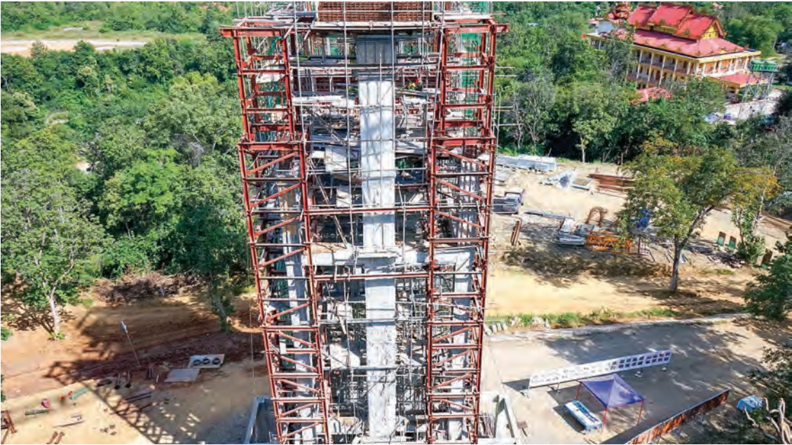
The elevator tower is 210 feet in length and 119 feet high. The tower also includes a 12-foot-wide walkway. The total cost is estimated to be about K1.6 billion. PHOTO: MAUNG MAUNG (MINBU)
