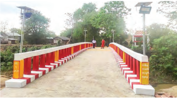
A concrete bridge repair work reaches completion.
