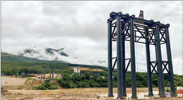
Construction site of the Kunlong Bridge.
