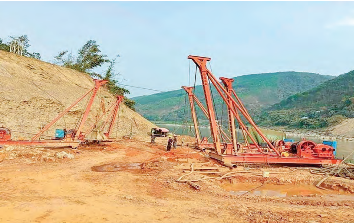
Foundation work is underway.
