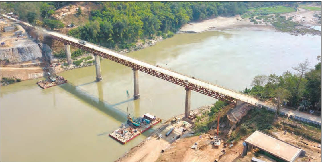
The bridge will be 351 metres long (1,151.631 feet), 39.4 feet wide (27 feet 10 inches wide for carriageway, 5 feet 9 inches wide for a sidewalk on each side) with a load capacity of 75 tonnes, and is made of a steel truss with reinforced concrete floor.
