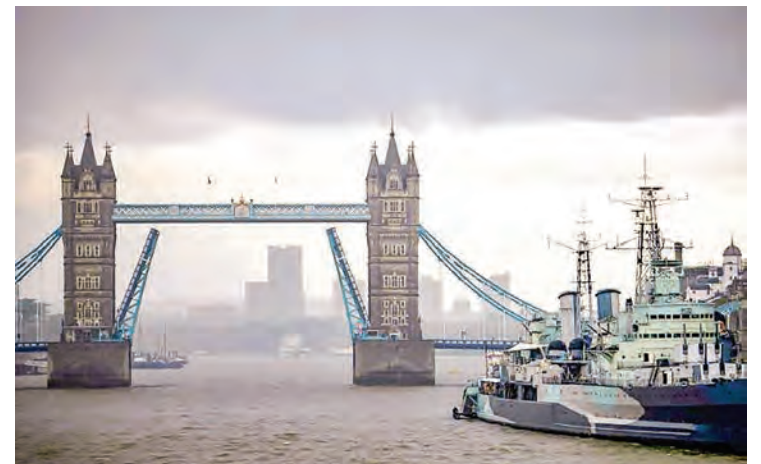
London's Tower Bridge is stuck in an open position due to a technical fault. PHOTO: AFP
