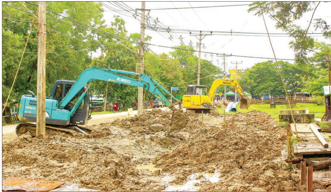
Heavy machinery are used in construction of water treatment plant in Dala Township to supply 3.3 million gallons of drinking water per day to local people.
