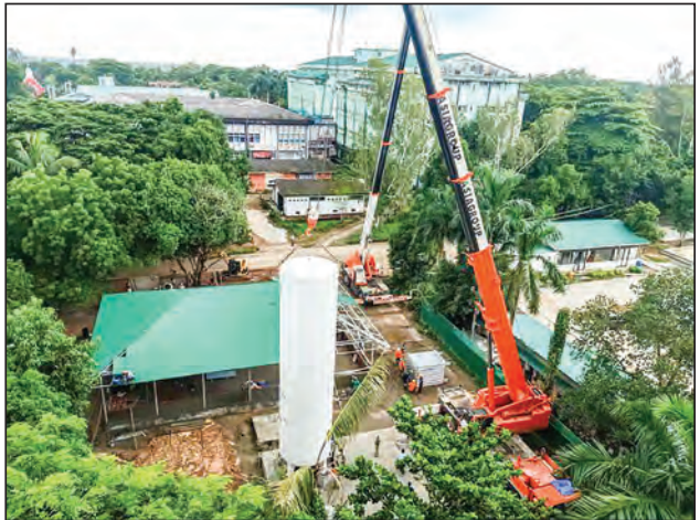
The work is underway day and night to complete the construction of a 30x30 feet plinth for the Oxygen Tank and 60x40 feet Filling Station by the end of this month.
