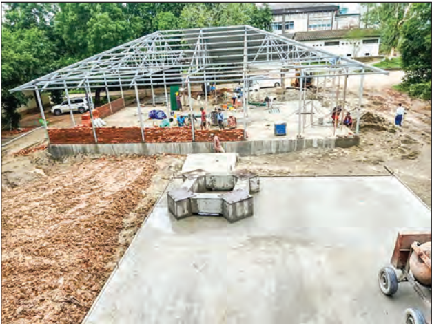
The work is underway day and night to complete the construction of a 30x30 feet plinth for the Oxygen Tank and 60x40 feet Filling Station by the end of this month.
