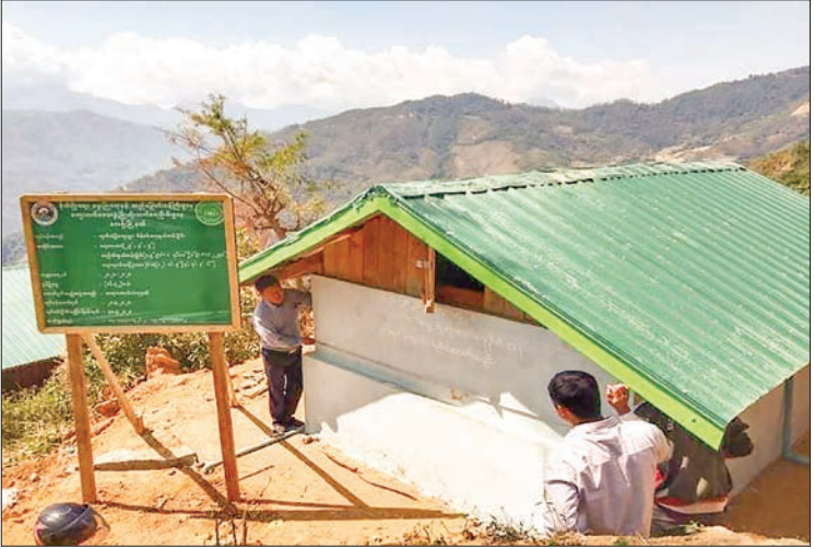
DRD carrying out to creat easy access of drinking water for the rural people.
