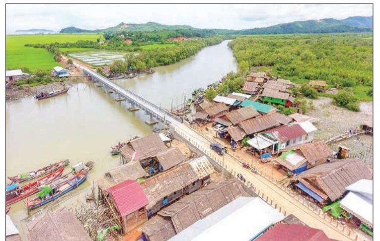
The 420-foot Pitat bailey bridge on the Pulaw-Laku-Myadaung Road.
