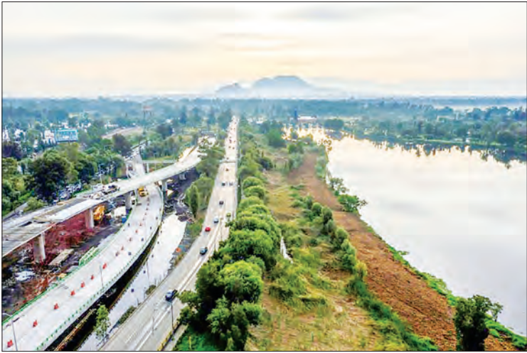
Activists fear a bridge being built over Mexico City’s wetlands will cause irreparable damage to the ecosystem. PHOTO: AFP
