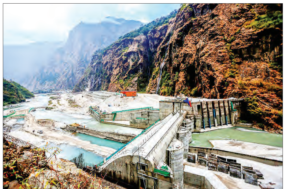
The project on Tamakoshi River in Dolakha district in central Nepal, approximately 200 km from the capital of Kathmandu, is one of the country's National Pride Projects. PHOTO: KATHMANDUPOST/XINHUA
