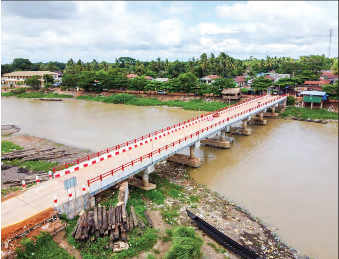
The concrete bridge, with a bored pile foundation, has a load capacity of 30 tonnes. The bridge is 260 feet long and 18 feet wide. The bridge clearance is 9 feet.
