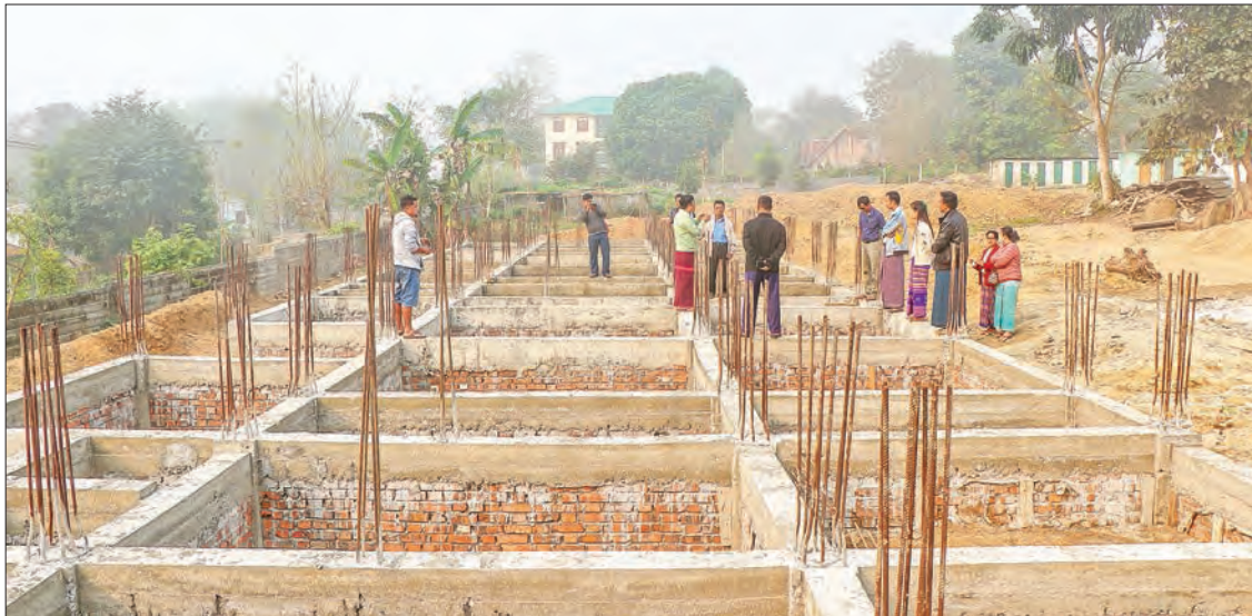
The housing quarter is a two-storeyed RC building, and it is 120 feet in length and 130 feet in width.
