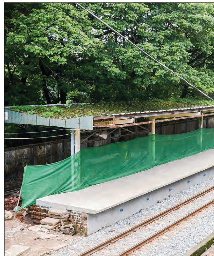
The platform at the Mahl wagone station is begun upgrading. (6459)
