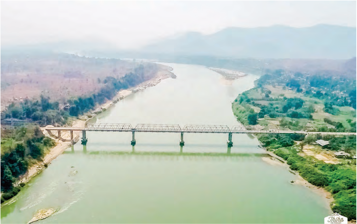
Thanlwin Bridge (Pasawng).
