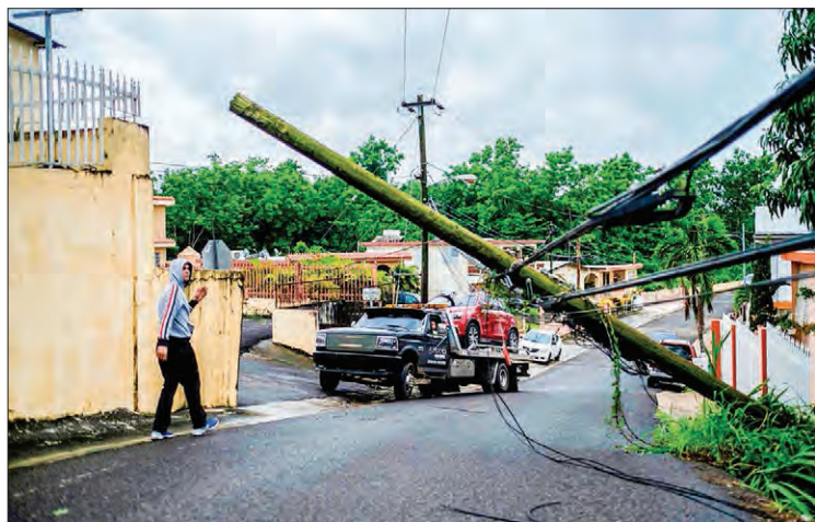
A man guides a tow truck under a downed power line pole after Tropical Storm Isaias affected the area in Mayaguez, Puerto Rico on July 30, 2020. (PHOTO BY RICARDO ARDUENGO/AFP)
