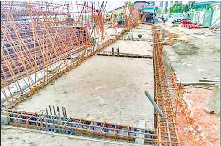
A line of concrete foundation is seen at Pathein jetty upgrade project i.
