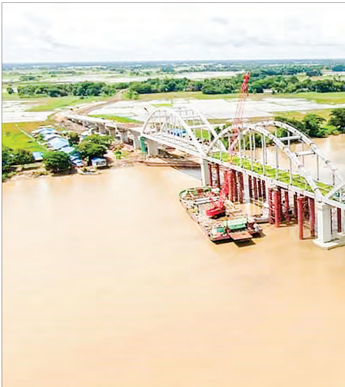
Kyunpyathat Bridge is a steel box girder with the floor of reinforced concrete and can withstand up to 60 tones of weight. —(Photo: IPRD)
