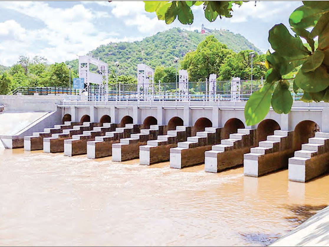
A dam gate is seen in Kyaukse Township, Mandalay Region. PHOTO: THET MAUNG (DISTRICT-IPRD)
