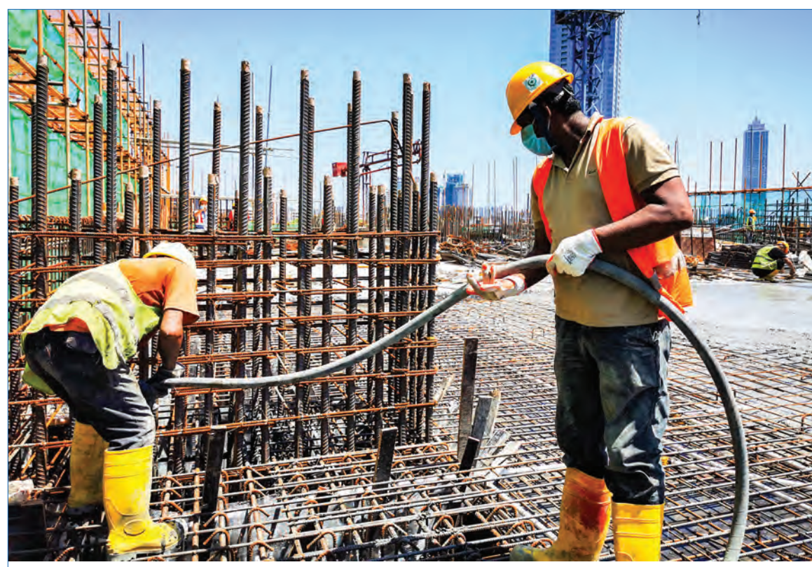
Photo taken with a mobile phone shows workers brought back to work by a tailored bus service at a construction site in Colombo, Sri Lanka, June 13, 2020. PHOTO: XINHUA
