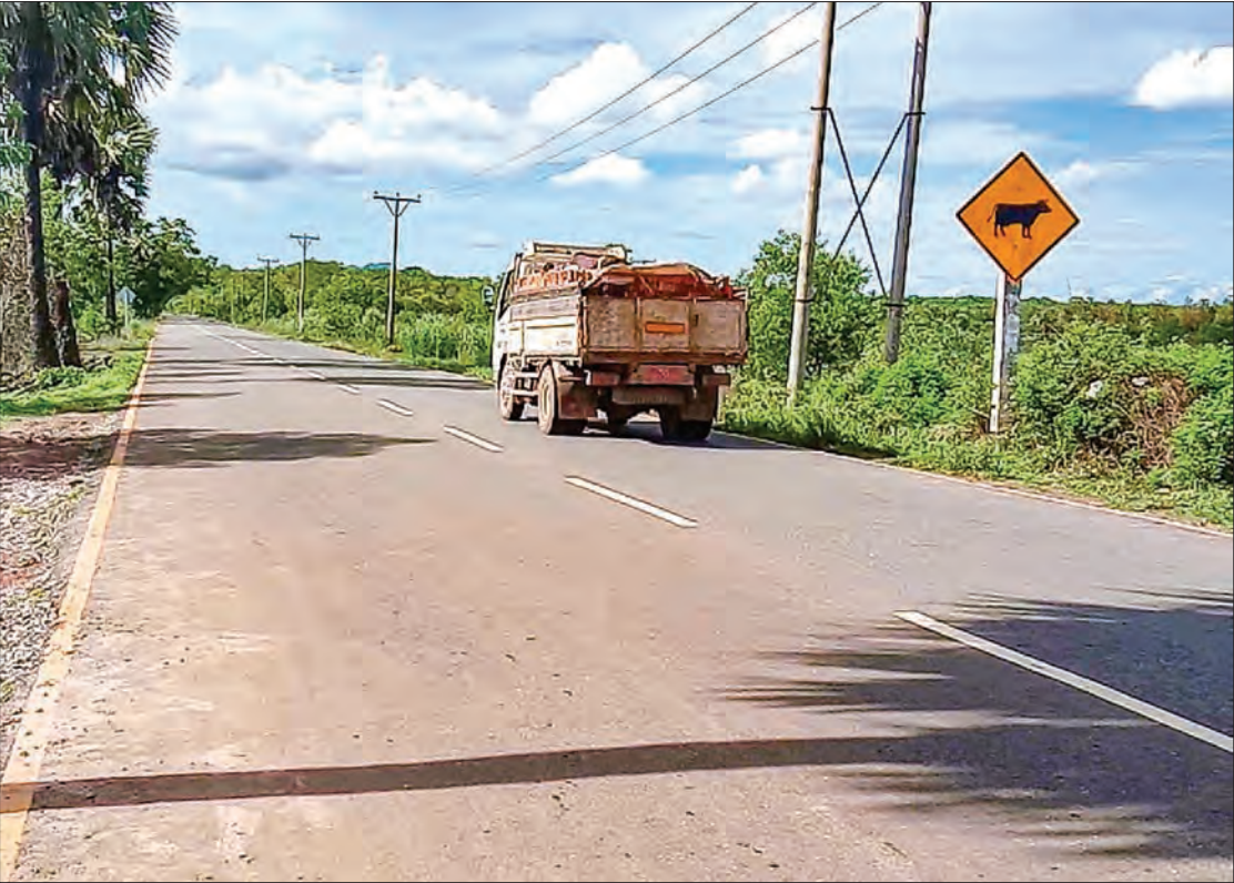
About 2,000 vehicles run on the Eindu-Zarthabyin road section every day, and its efficiency is expected to increase after bridges on this road are complete in 2023. PHOTO: SAW MYO MIN THEIN (IPRD)
