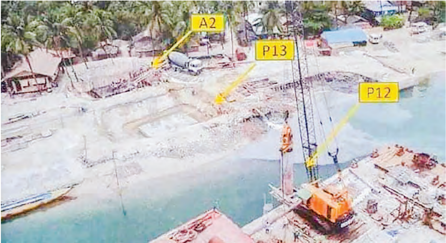
Photo shows construction site of the Gwa-Makyayngu Bridge being built with the use of heavy machinery.—(Photo: IPRD)
