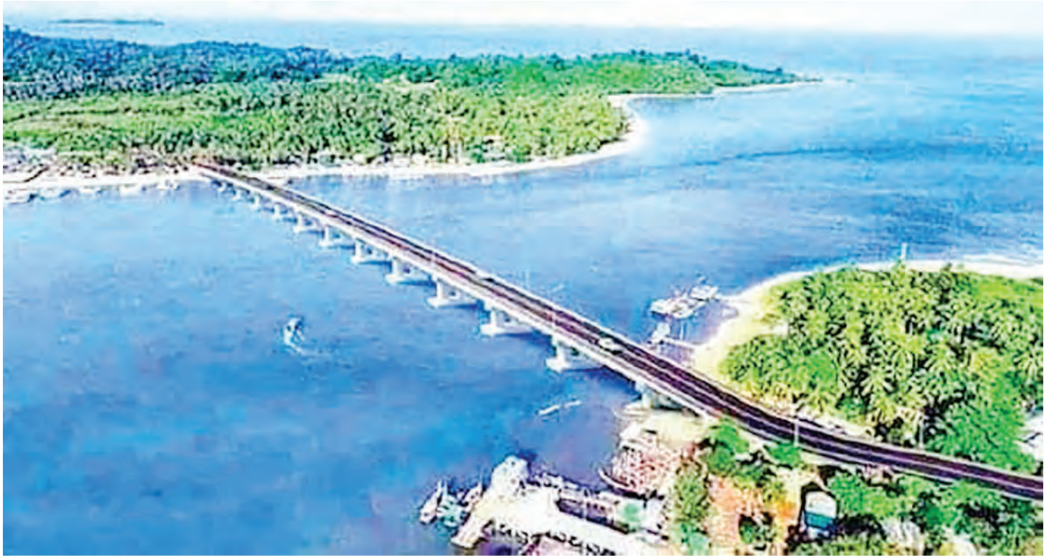
The Gwa-Makyayngu Bridge under construction in Gwa Township will connect Ayeyawady Region and Rakhine State.—(Photo: IPRD)
