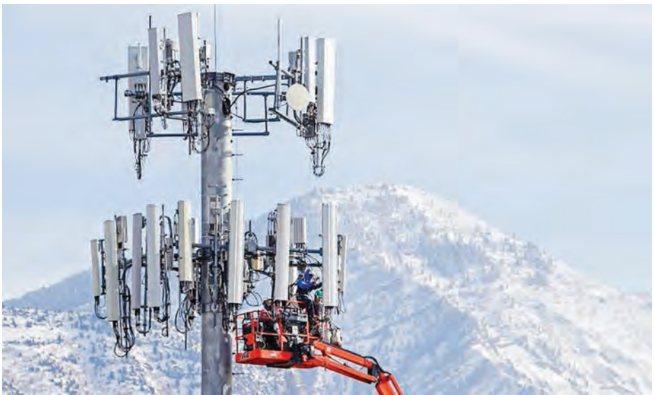
A Verizon crew updates cell tower equipment for the new 5G network in Orem, Utah. PHOTO: AFP
