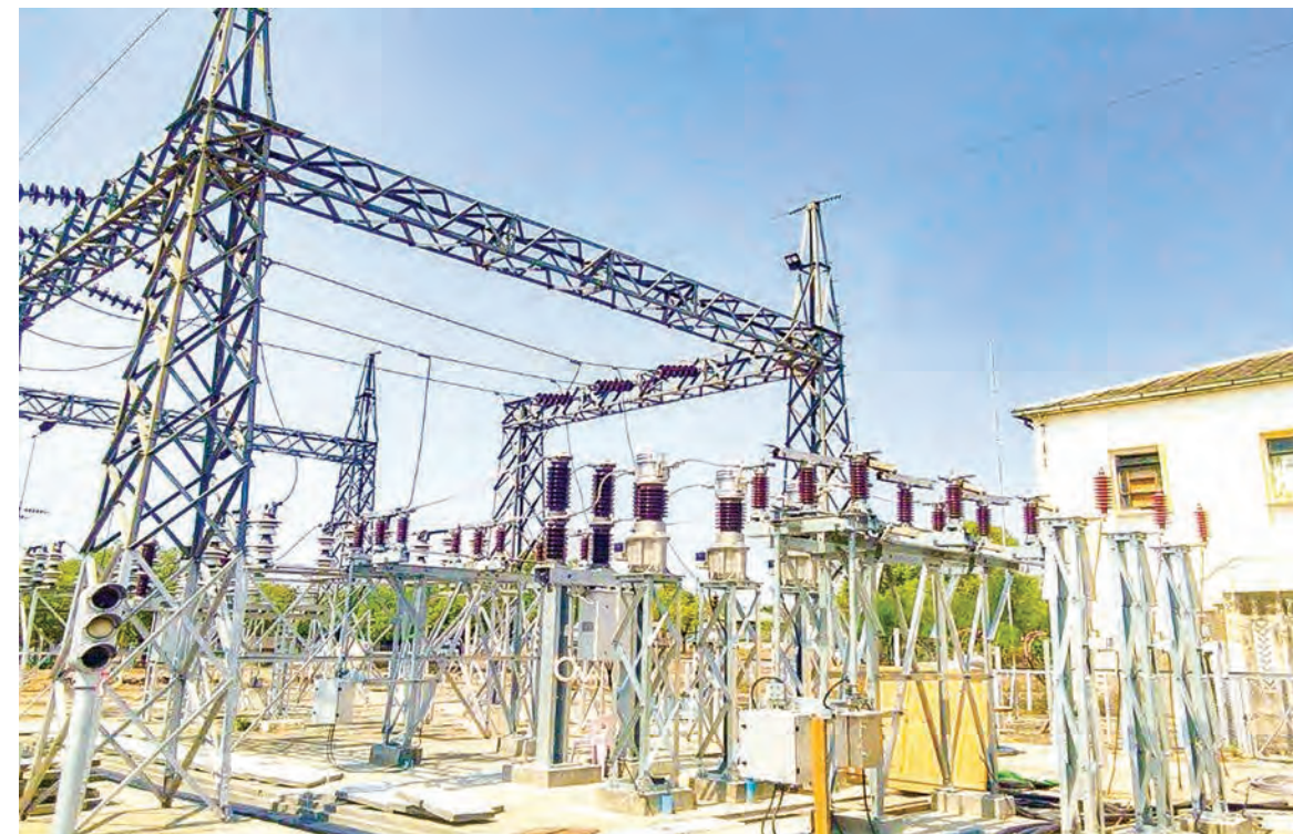
The 33KV Switchbay of Mandalay's Thazi Sub-power station.
