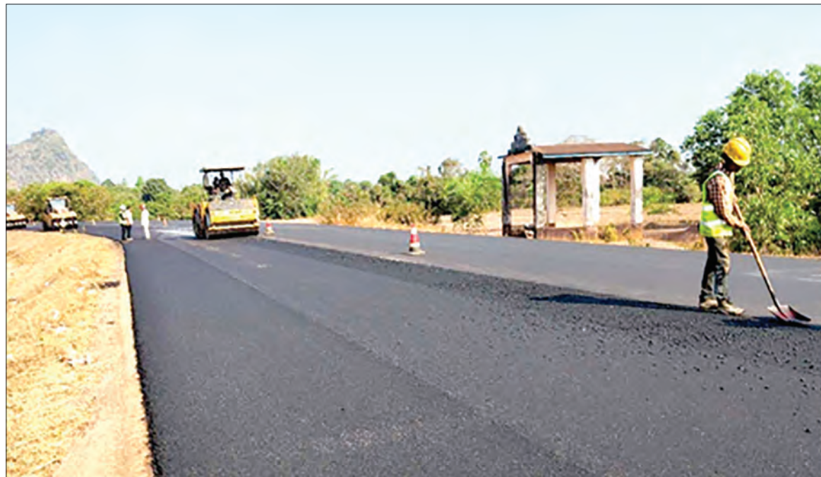
Eindu-Kawkareik Road is being upgraded on 5 Nov 2019.
