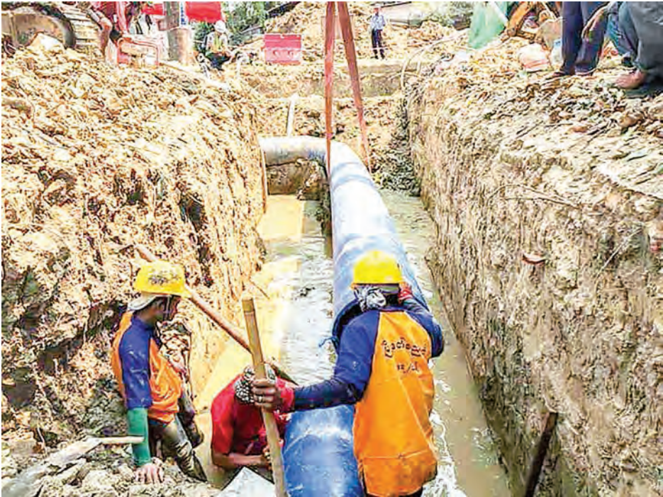
Yangon City Development Committee’s workers laying water pipeline to the Eco Green City.
