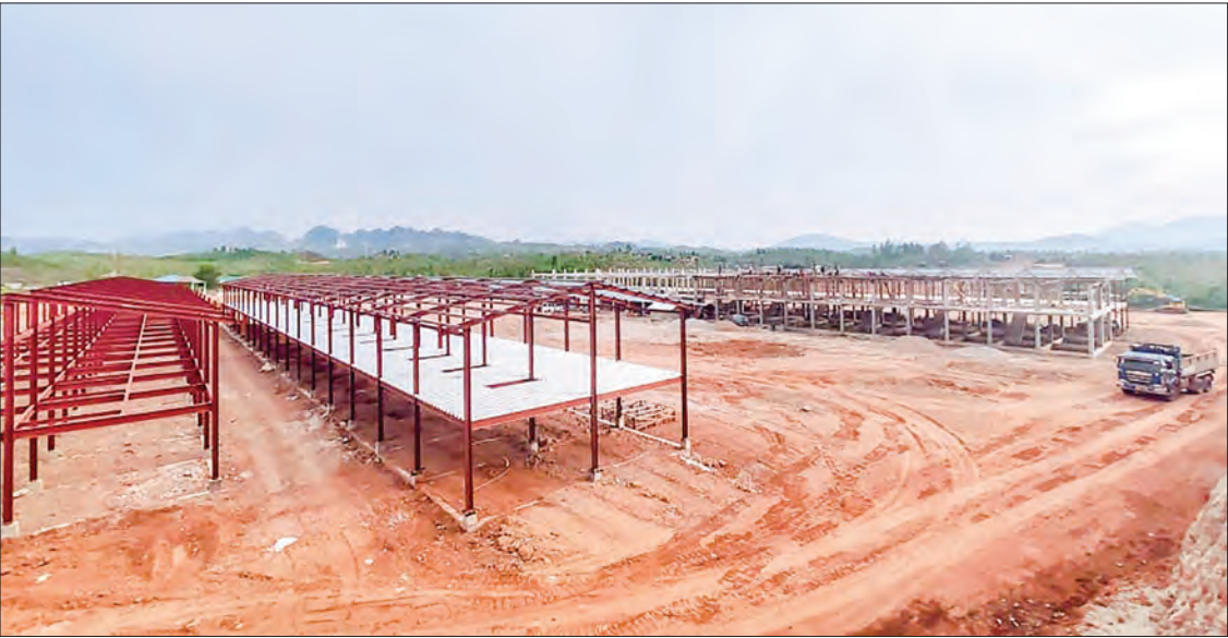
The construction of Myawady highway bus terminal is underway. PHOTO: HTEIN LIN AUNG (IPRD)
