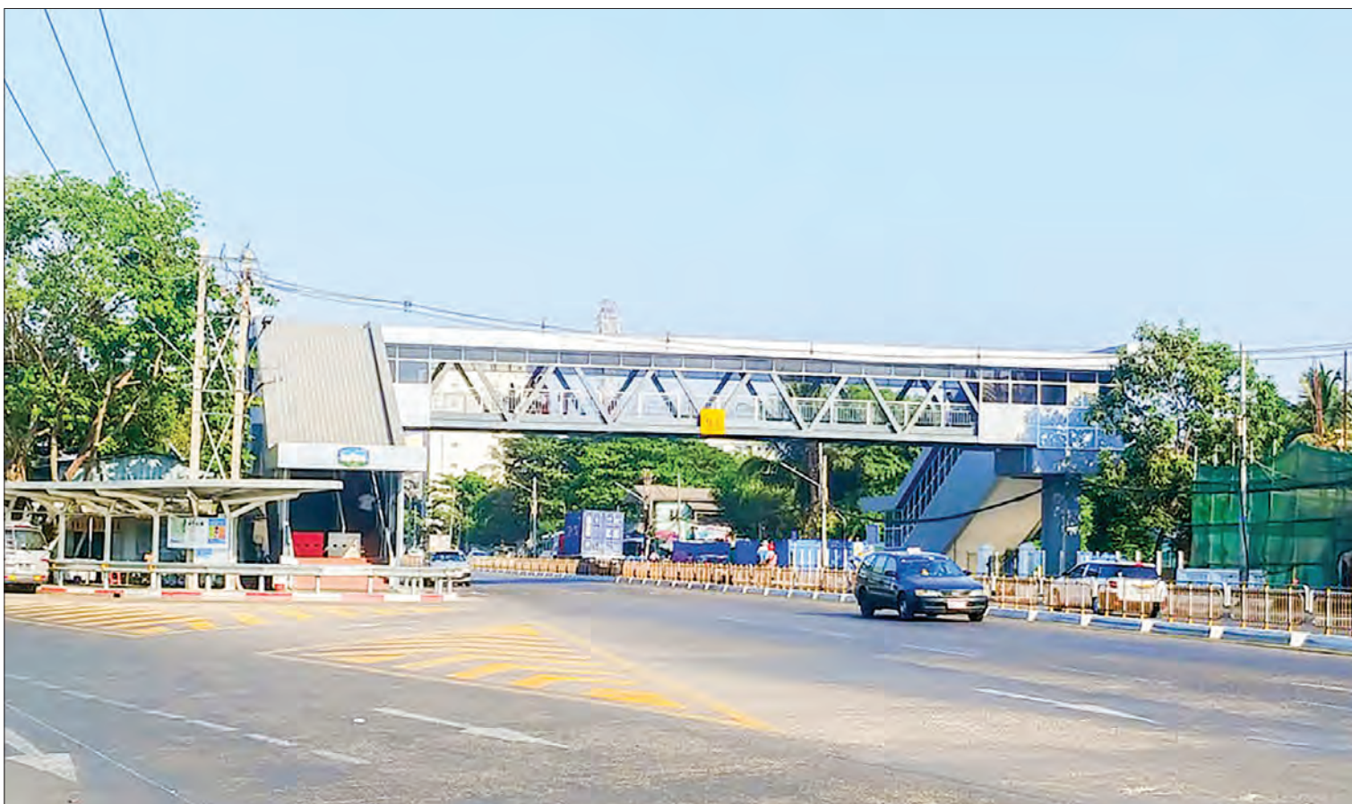
Dawbon pedestrian overpass. PHOTO: AUNG YE THU (DAWBON)
