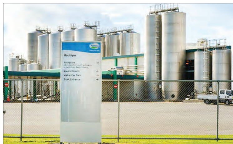
Fonterra's Hautapu dairy factory, located near the rural town of Cambridge, some 150 km south of New Zealand's largest city, Auckland. PHOTO: AFP
