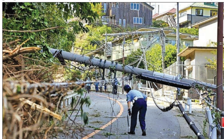
Experts accuse the Japanese government and utility companies of being unprepared as tens of thousands of homes were still without power nearly two weeks after Typhoon Faxai hit. PHOTO: AFP
