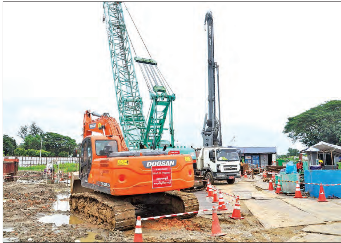
Bored piling machine in operation at the construction site of the new bridge linking Thanlyin and Thakayta. PHOTO: THAN SOE
