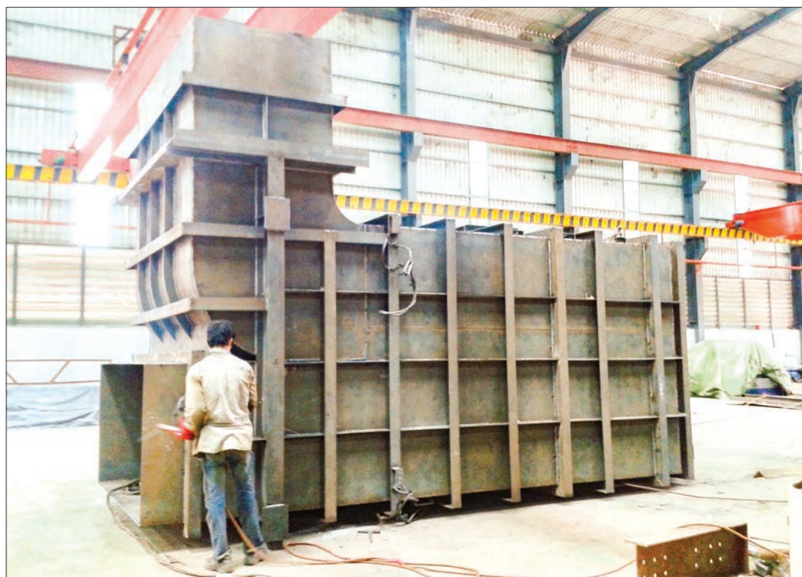
Fabricating a factory smoke stack. PHOTO: SIM
