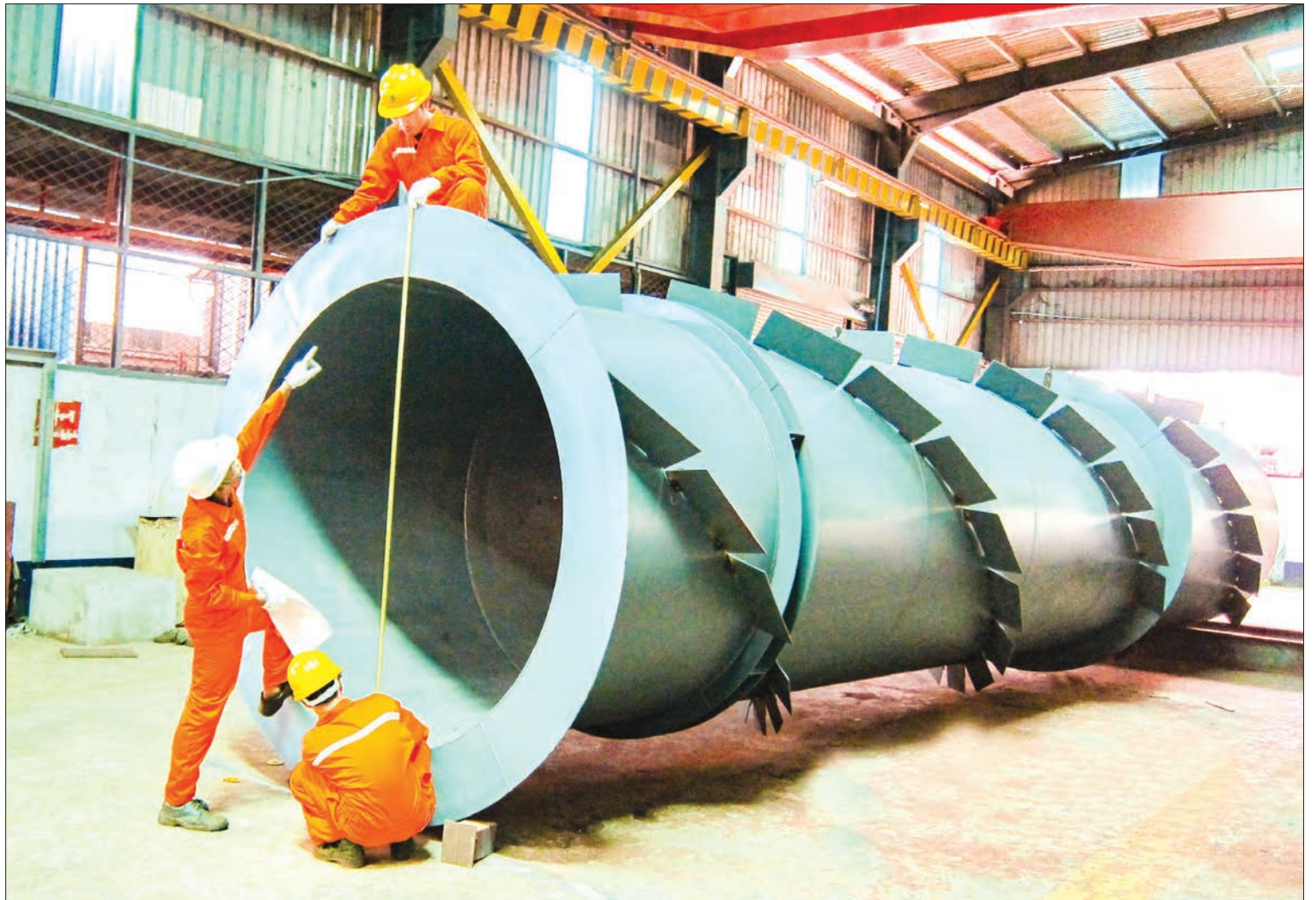
Fabricating a factory chimney. PHOTO: SMI
