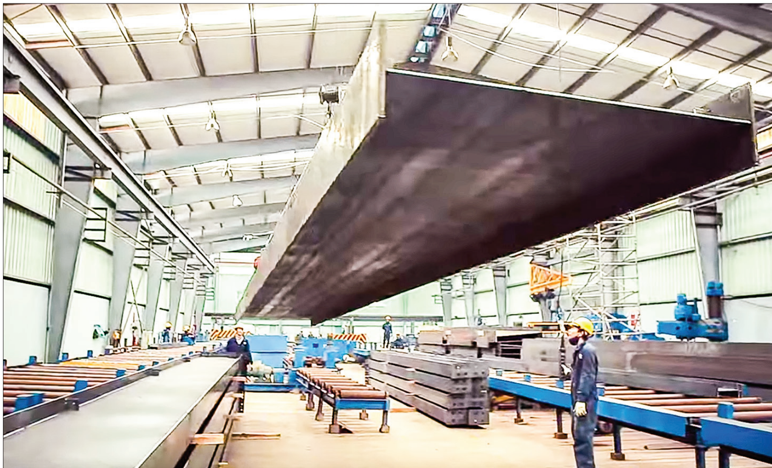
Workers moving steel beams. Photo: Supplied
