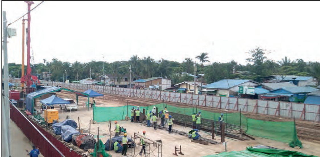
Workers being seen at the construction site of Yangon-Dala bridge. PHOTO: MAUNG YIN OO(DALA)
