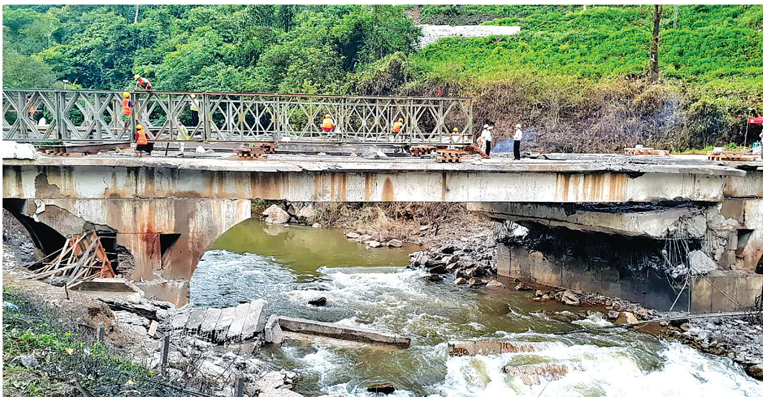
The Special Bridge Construction Teams are building a 210 ft-long bailey bridge to replace the Gote Twin Bridge in Nawngkhio. PHOTO: MNA
