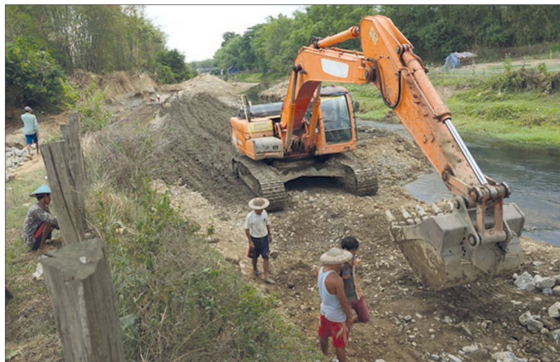
A retaining wall is being built in Mohnyin Township, Kachin State with the use of heavy machinery. PHOTO: SUPPLIED
