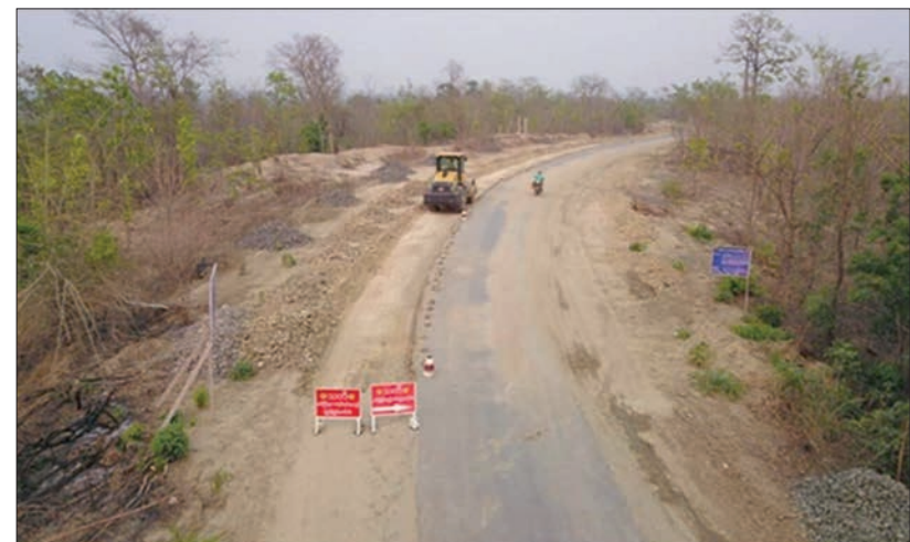
The Shwebo-Myitkyina Road linking Sagaing Region with Kachin State is being extended to 18 ft wide from 12 ft wide. PHOTO: SUPPLIED
