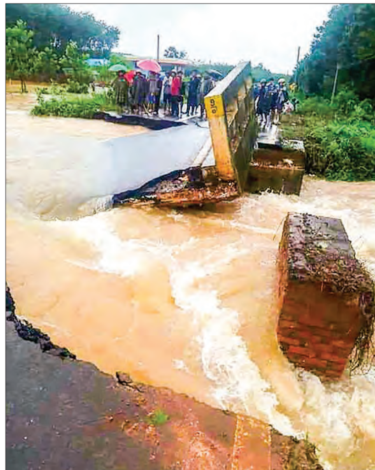
Flood damages the concrete bridge in Kyaikmaw on 9 August. PHOTO: CHO MYAT HTWE (KYAIKMAYAW)
